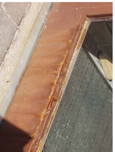
Centre window & door frames rusted
